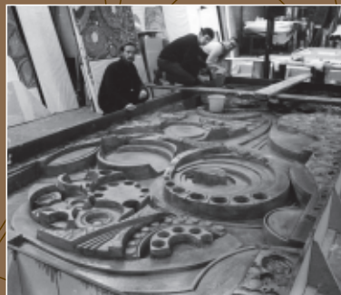
New County Buildings Paisley. In the Studio/Workshop. Moulds for fibreglass relief mural. Size approx. 8 ft high and 20 ft long. Architect: Hutcheson, Locke & Monk Architects. c.1971
